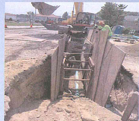
Sewer pipe replacement across Nantasket Avenue
